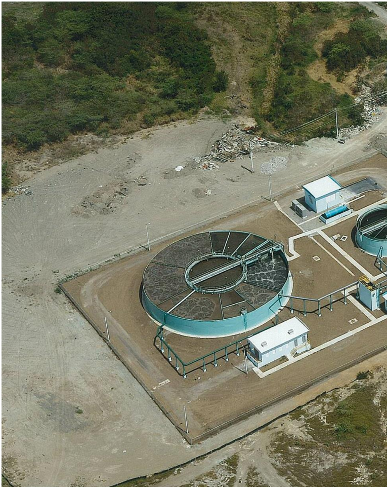
WWTP Expansion Guanica
