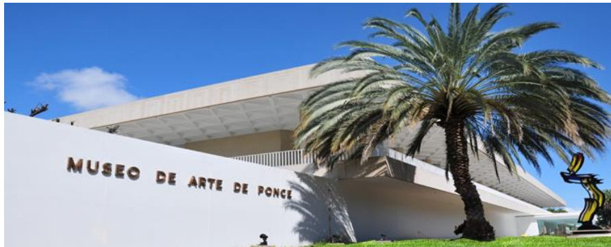
Museo de Arte de Ponce Annex Building: Project Management
